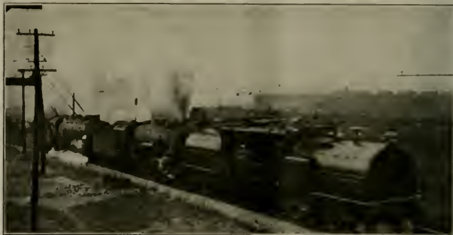
TESTS OF GEARLESS LOCOMOTIVE. STEAM AND ELECTRIC LOCOMOTIVES DURING REGENERATIVE BRAKING TEST.
